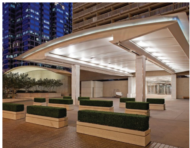
Figure 1-1. Bright porte-cochere lighting announces building entry and provides a sense of arrival.
